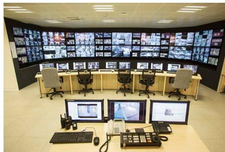
*Airport security staff can view the airport's CCTV, access control, fire safety systems and also intrusion systems from the central control room.*
